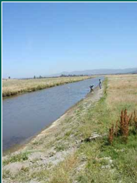
Pre-restoration condition in the SWOA, June 2001.
