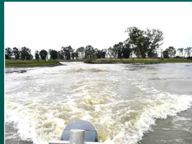
SWOA levee breach, March 2004.
